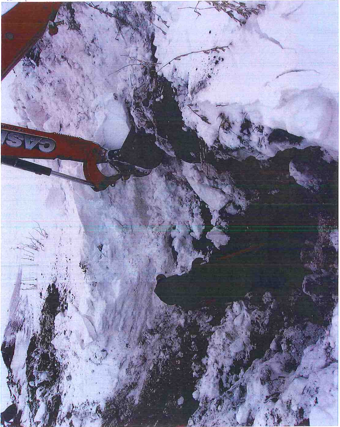
REMOVING SNOW FROM EXISTING HOLE @ #340
