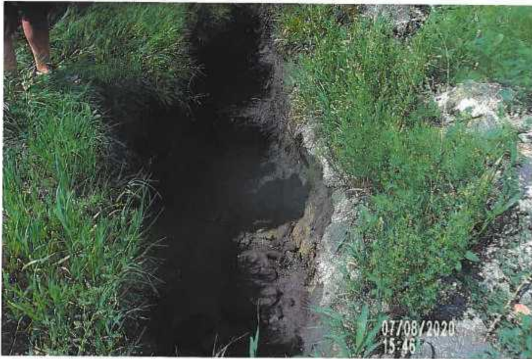
PICTURE#4067 IS LOOKING NORTH SHOWING PREVIOUSLY EXCAVATED HOLE EAST OF EAST ROW FENCE FOR CO. HWY 527 & SOUTH OF CO HWY D41
