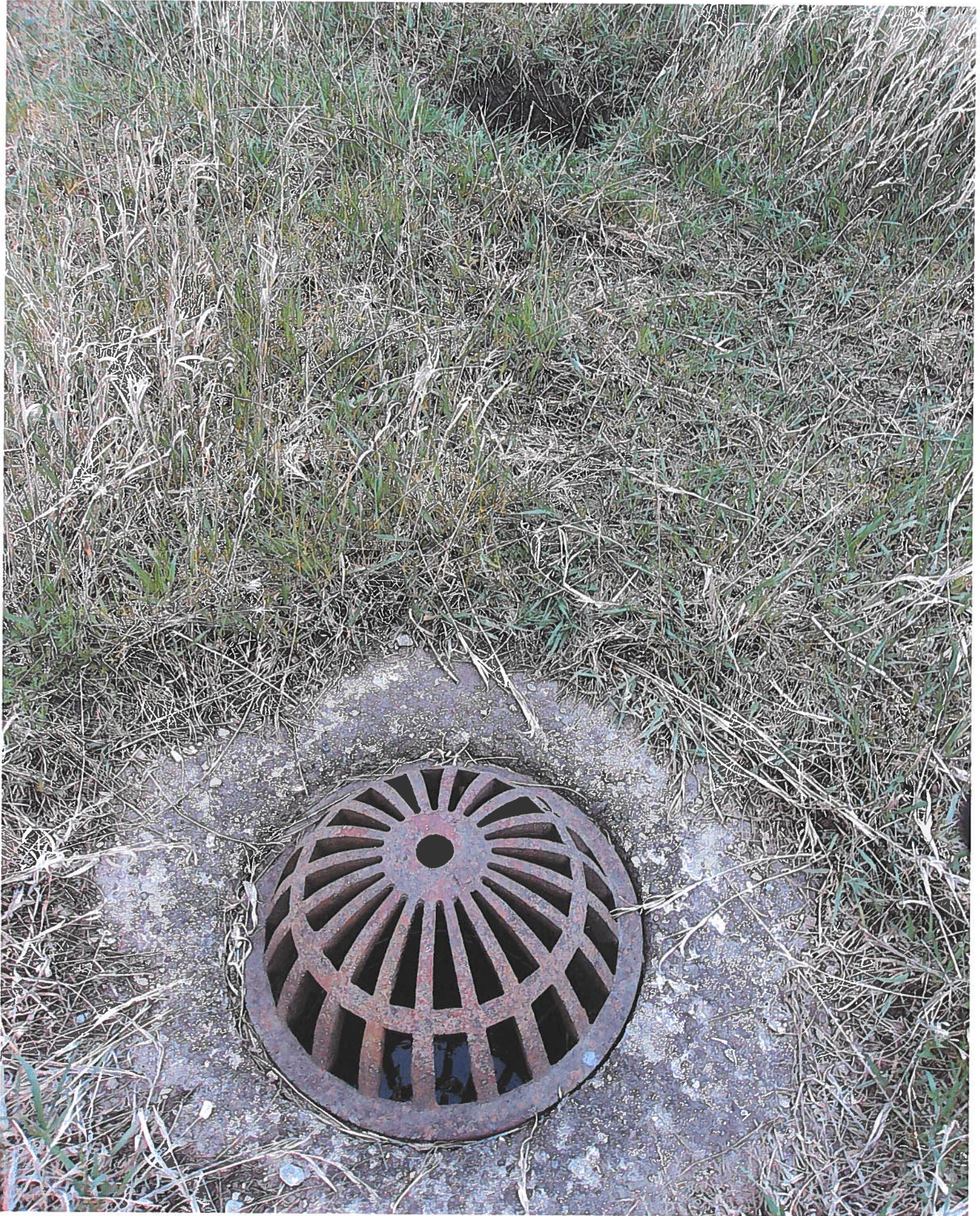
LOOKING EAST @ BEEHIVE WITH HOLE ON LAT2, S. SIDE D41 BY CRP
