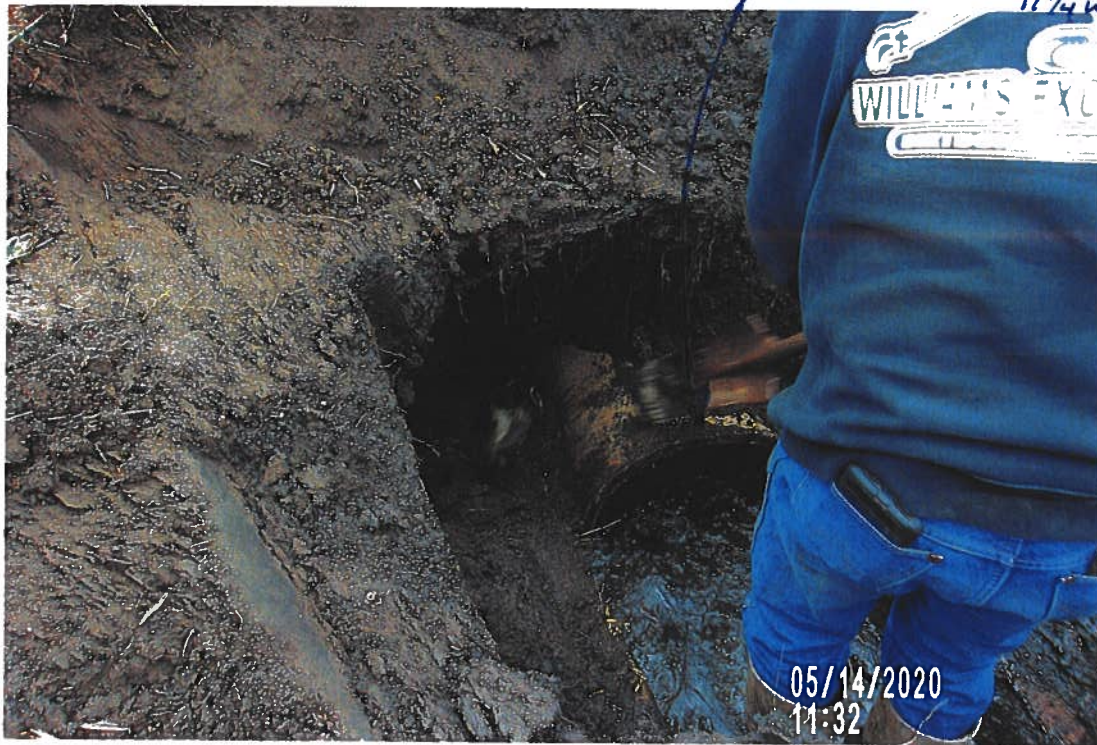
PICTURE #354D IS LOOKING SW IN BLOWOUT #2S SHOWING 5.5' LONG ERODED SOIL CAVITY ON EAST SIDE OF TILE
