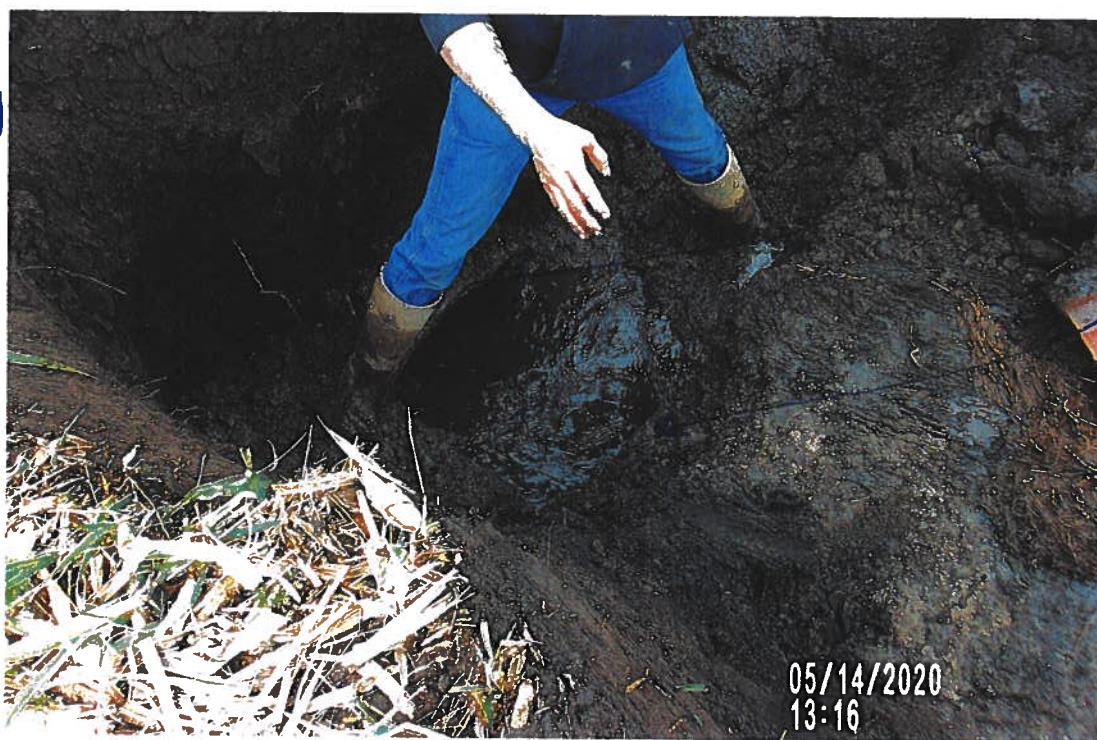
PICTURE # 3553 IS LOOKING NE SHOWING COLLAPSED SECTION OF TILE REMOVED AND NOW FLOWING GOOD IN BLOWOUT. IN
