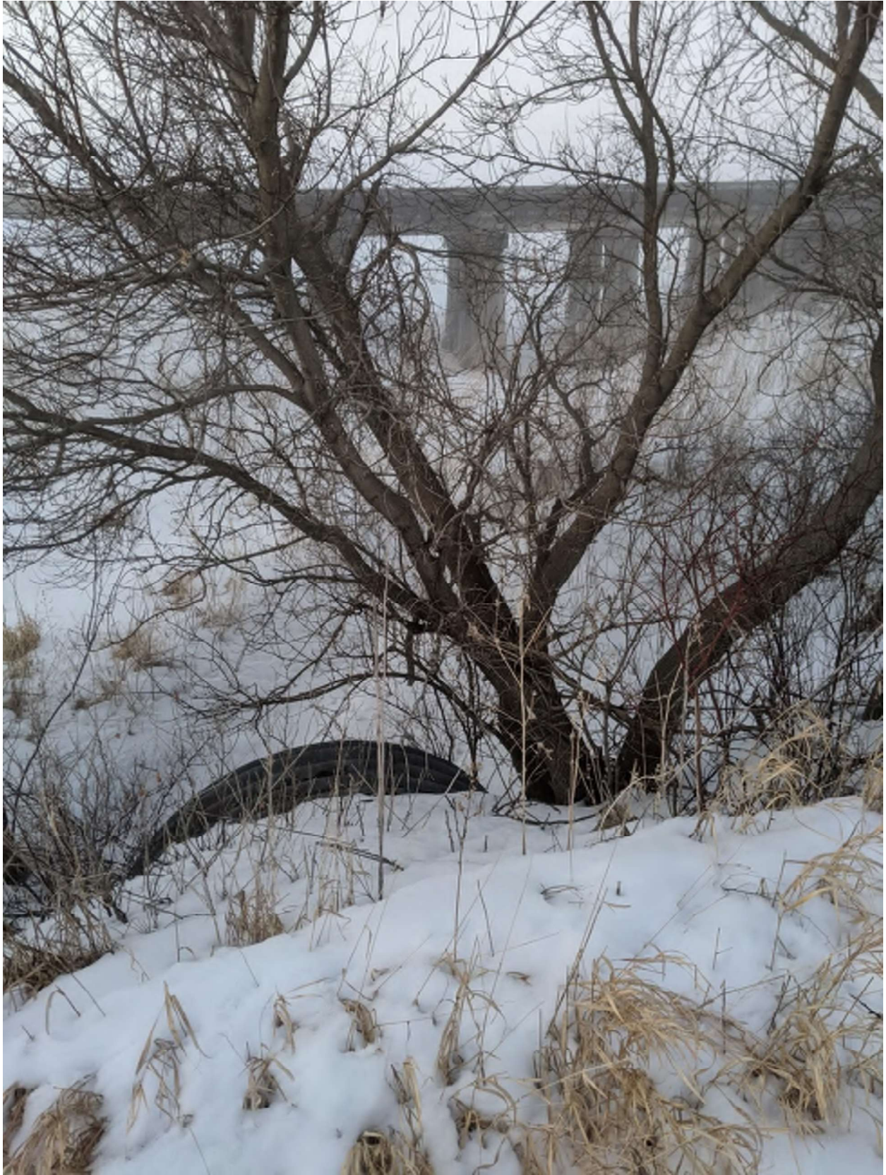
Figure 4: Large trees and woody brush growing over the lower 200 feet of both Main tiles.
