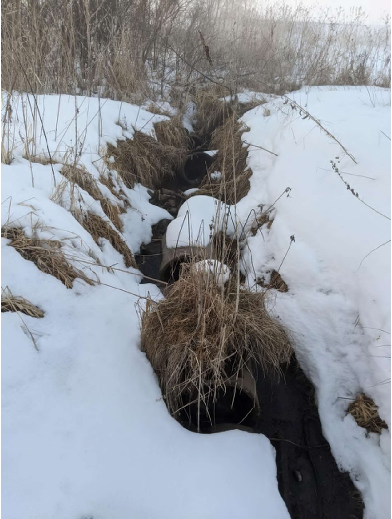
Figure 2: Lower 100 feet of 1922 Main.
