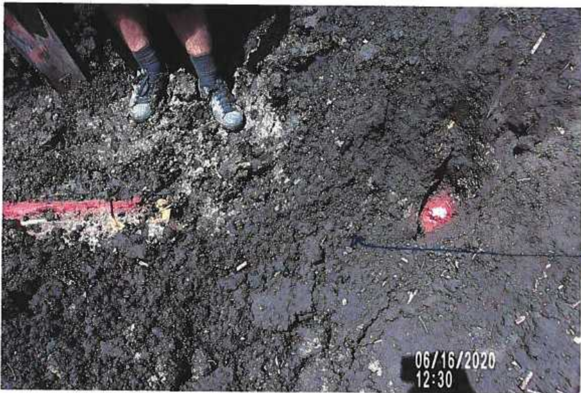
PICTURE #3777 IS LOOKING SLIGHTLY NW SHOWING EXISTING CLAY TILE TO SW IN GOOD SHAPE AND SECTION OF CLAY TILE COLLAPSED (GOOD CLAY AROUND TILE)
