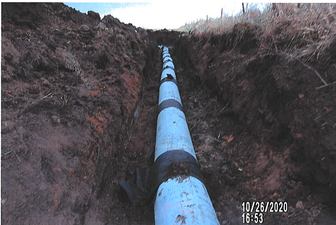
PICTURE# 4719 IS LOOKING EAST SHOWING TILE WITH JOINTS WRAPPED & SITING IN TROUGH FROM SPOON BUCKET EAST OF GPS # 7298
