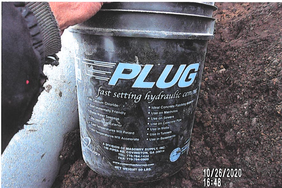
PICTURE# 4718 CREW USED THIS TO GROUT WIDE JOINTS ON 15" RCP TILE.
