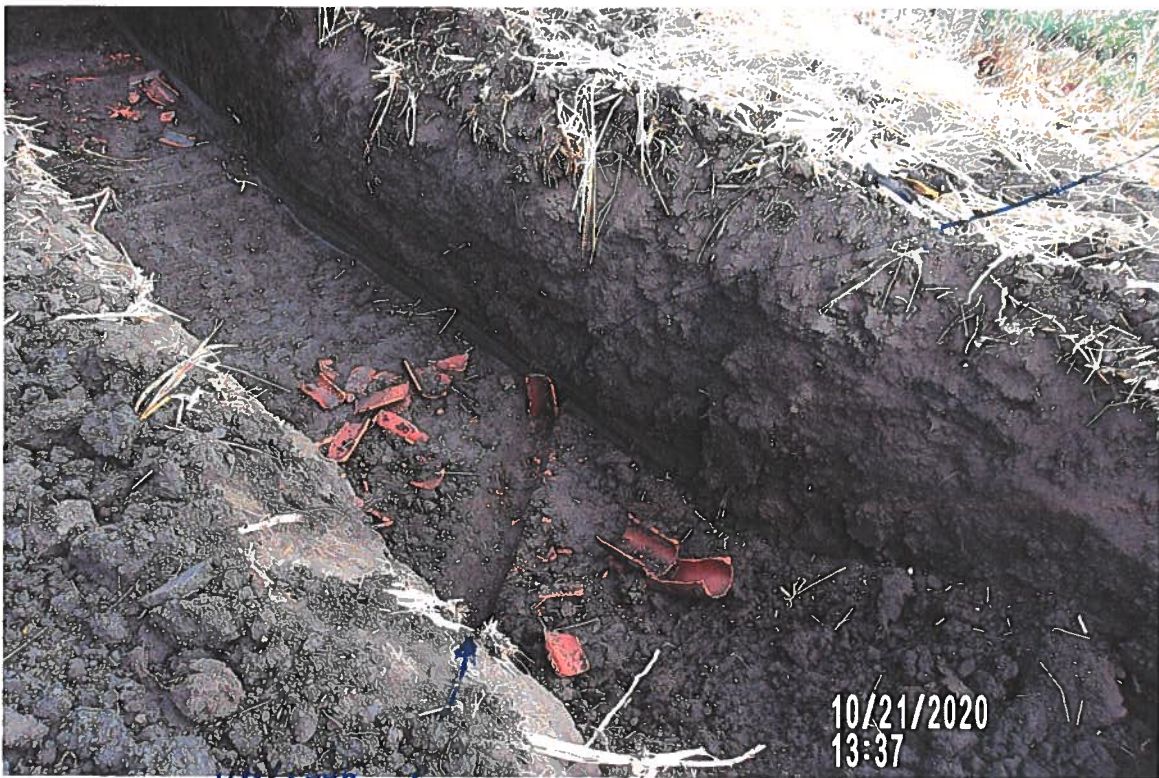
7" CLAY 4.4' DEEP 7275 PICTURE # 4688 IS LOOKING NE TOWARD MAIN TILE TIE IN SHOWING 7" CLAY TILE WITH CHUNK OF TILE BLOCKING DOWNSTREAM END.
