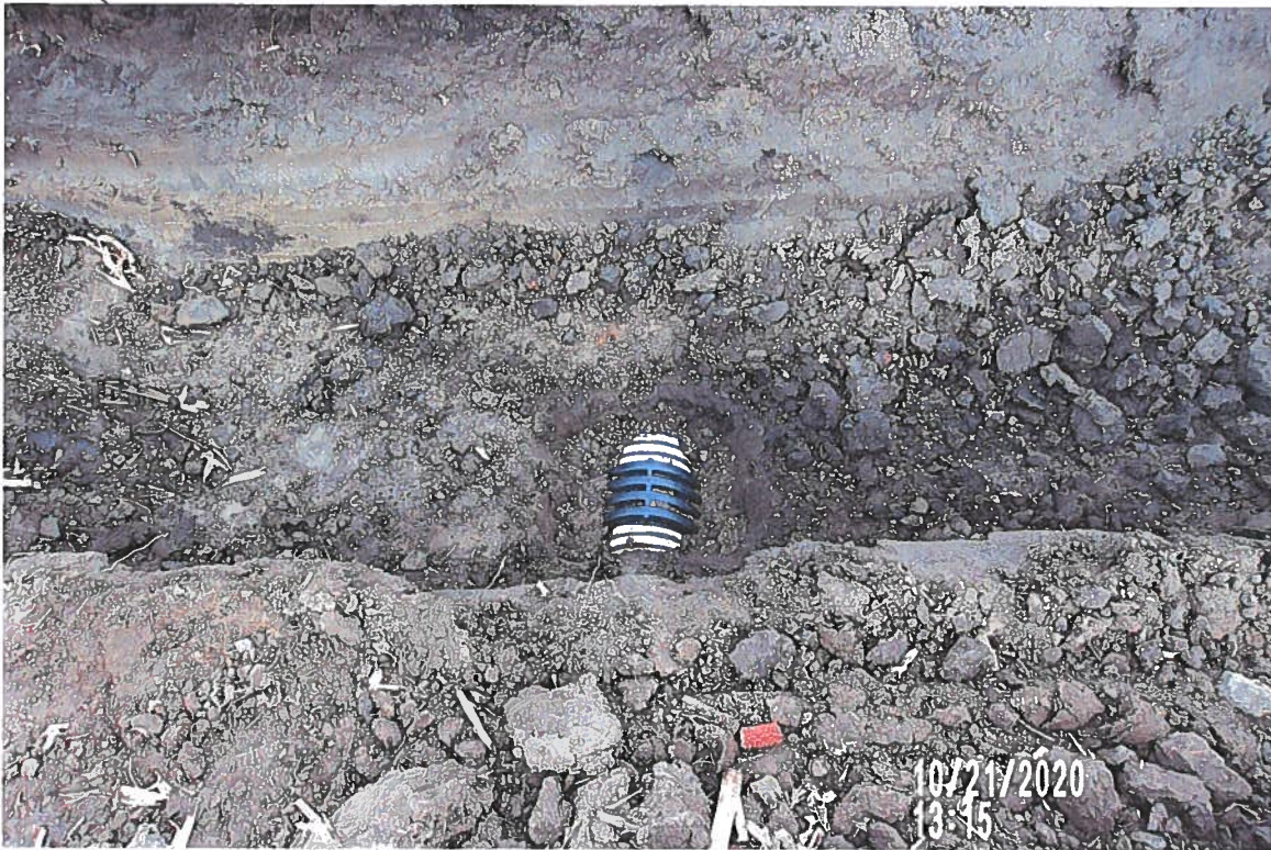
PICTURE # 4687 LOOK NORTH SHOWING CREW PLACED CHUNK PLASTIC TILE OVER HOLE IN TOP OF EXPOSED 8" PERF TILE @ GPS# 7249.
