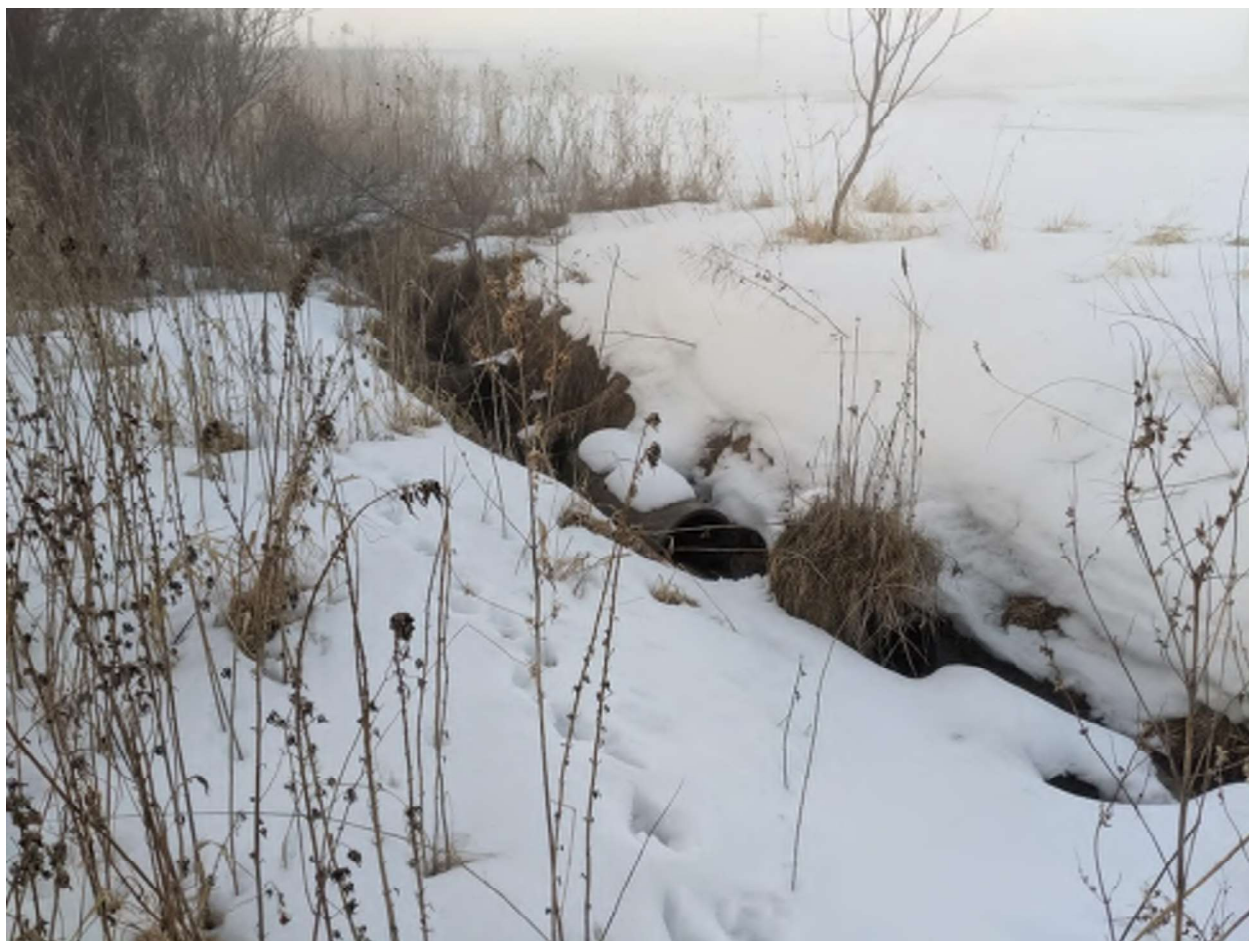
Figure 1: 1922 Main completely exposed and broken above outlet.
