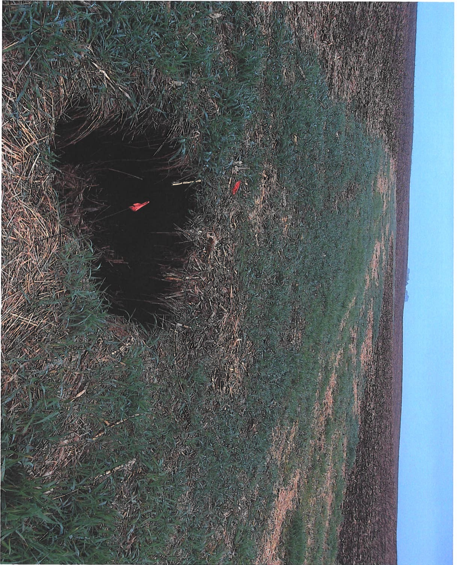
NORTHERN most Blow-out, COLLAPSED TILE 15" \phi \pm
