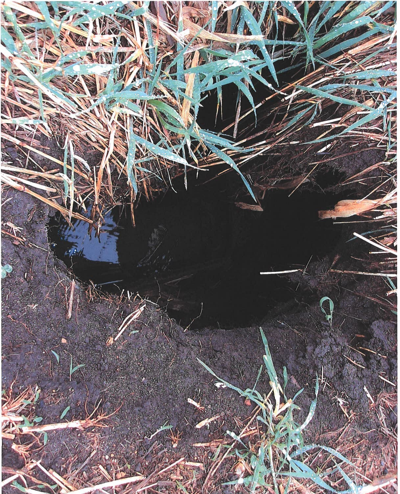
Collapsed Clay Tine
