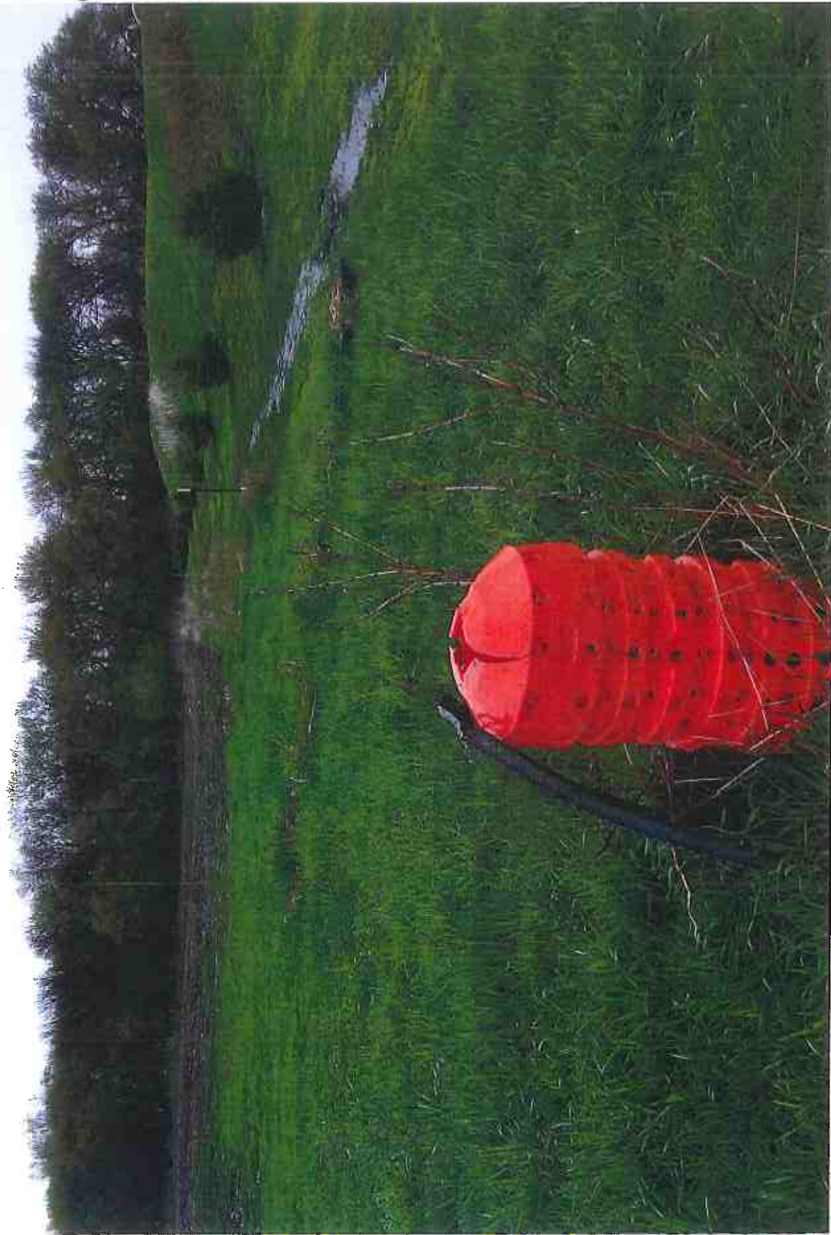
12" HICK INTAKE FULL OF WATER, SWIRLING
