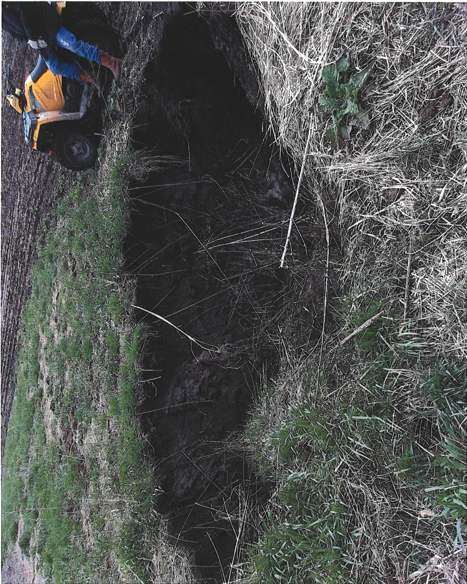
Blow-out Hole on DD 100, MEASURED 12" TILE
