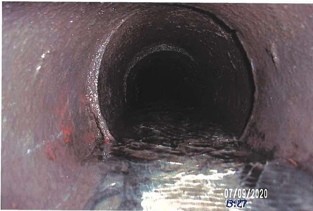
PICTURE #4103 IS LOOKING UPSTREAM INSIDE 8" CLAY TILE WITH ABOUT 1" FLOW AT GPS #302 (TOP 8" CLAY TILE) (0.72' TOP TO FL)
