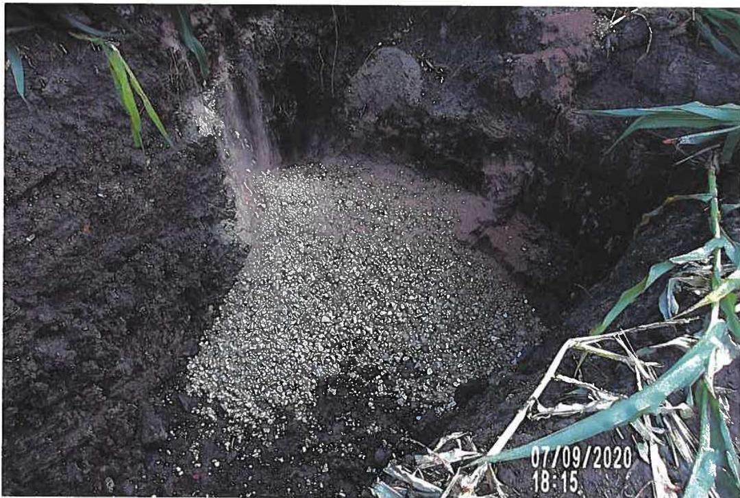
PICTURE# 4128 IS LOOKING NW SHOWING NORTH 14" CLAY TILE EXPOSED TRENCH WITH TILE BEDDED WITH ROCK TO TOP OF TILE
