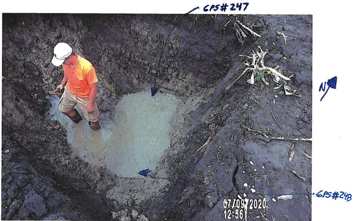
PICTURE #4101 IS LOOKING NW AT FINISHED 3/4 CONCRETE COLLAR FOR 14" CLAY TILE REPAIR 168'± NORTH OF E HWY D41. CREW USED 18-60LB QUIKRETE HIGH STRENGTH CONCRETE BAGS FOR CONCRETE COLLARS.
