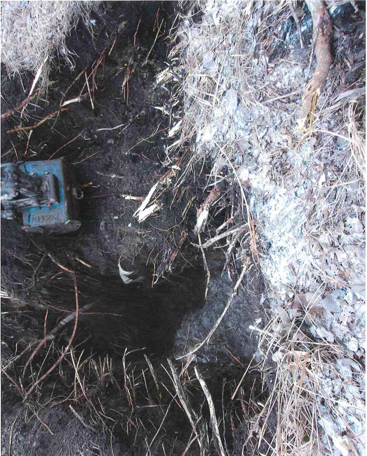
ROOT PLUG TAKEN OUT OF 12" CONC. TILE, WATER IS RUNNING LOW VOLUME, CONC. TILE IN GOOD COND.
